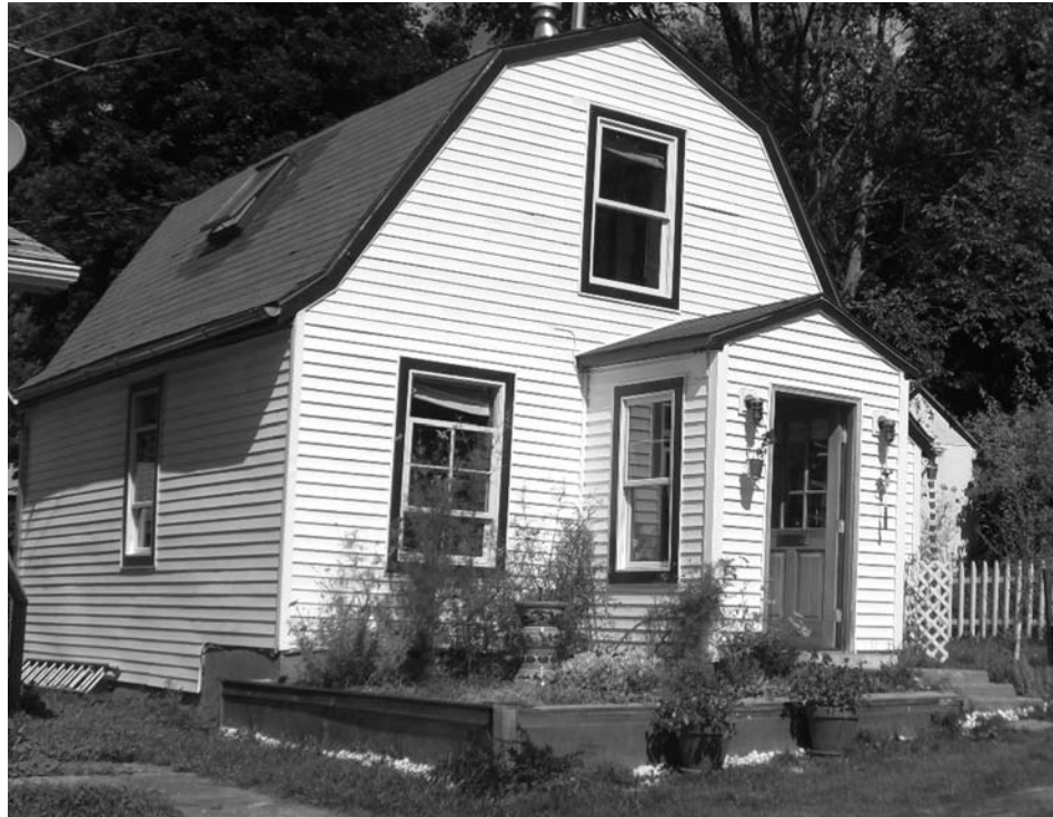
The outside after, above, and before, below.
